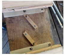
down, 25 mm screws at the top and 35 at the bottom.
